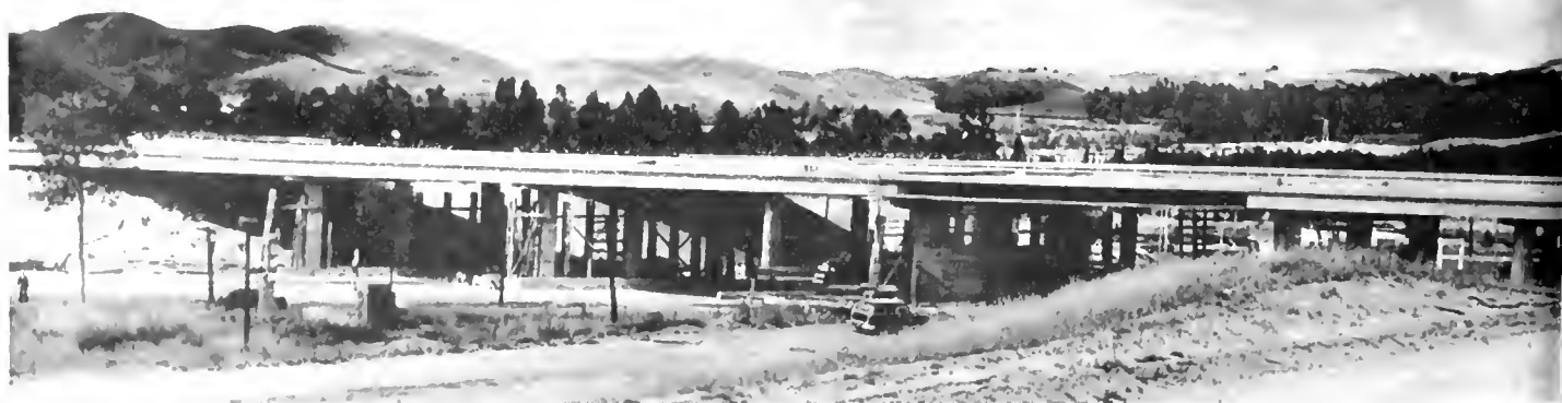
Looking westerly of Golden State Freeway bridges over San Fernando Road and the mainline Southern Pacific Railroad track
